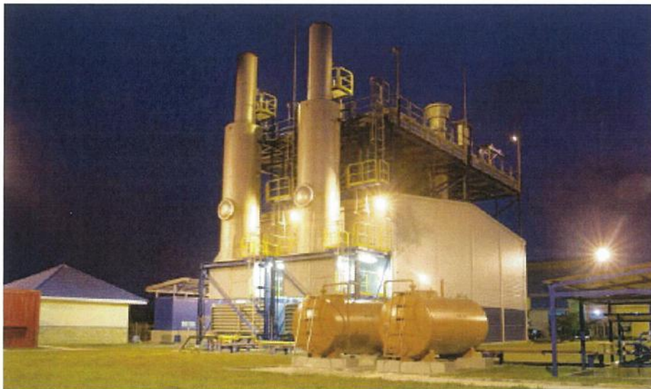
FIGURE 5.1-3 : BOIL-OFF GAS POWER PLANT (W16V34SG)
