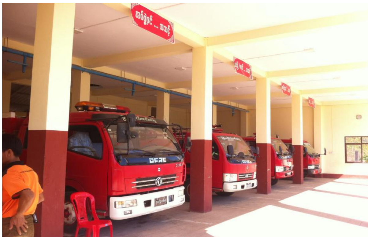
Figure 4.1-48 Yebyu Fire Station and facility in Yebyu Township
