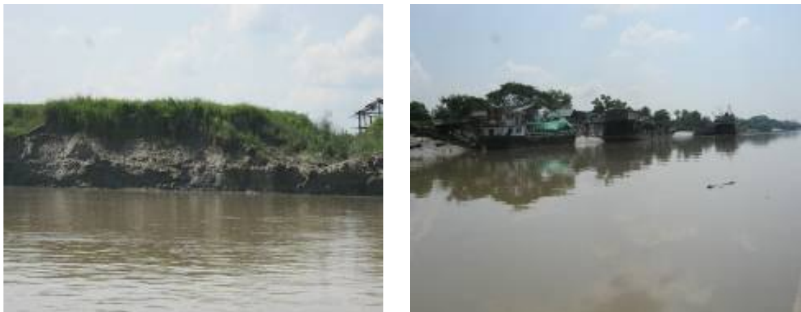
Figure 5.2-24 SW13: River Bank Erosion and Small Port Activity
