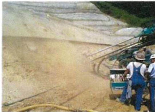
Soil Nailing Construction Techniques
