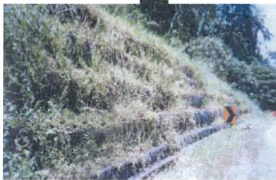
Gabion Wall Together with Grassing
