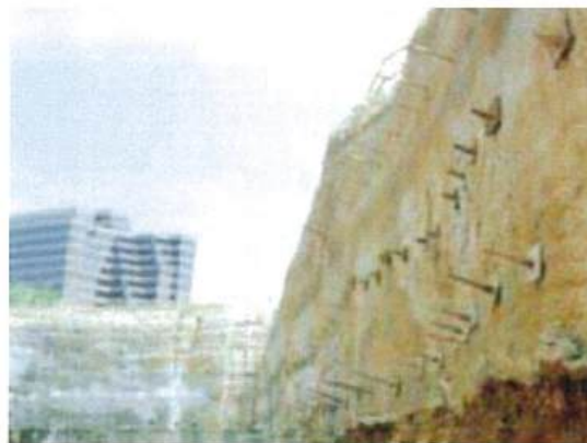
Soil Nailing Application
