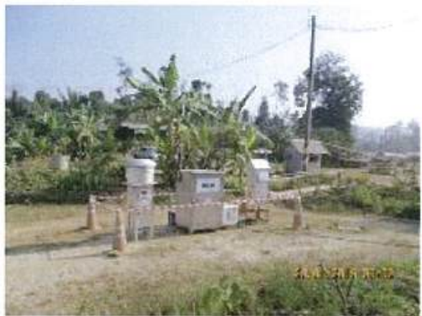
Equipment for Wind and Air Quality Data Collection at Station 3: Elasto Base 1 Camp
