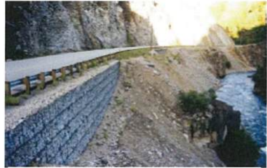
Gabion Retaining of Side Slope
