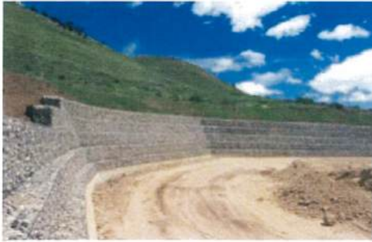
Gabion Retaining Wall of Back Slope
