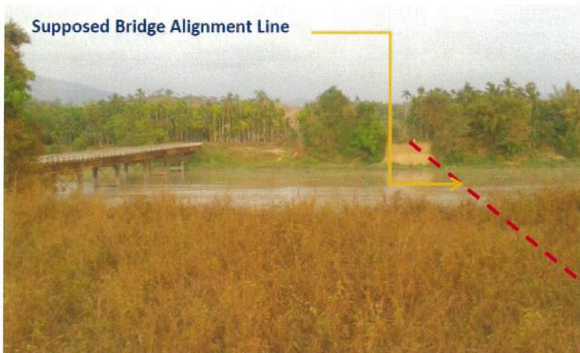
PHOTO 4.2-1 : DAWEI RIVER AT STA.16+885
